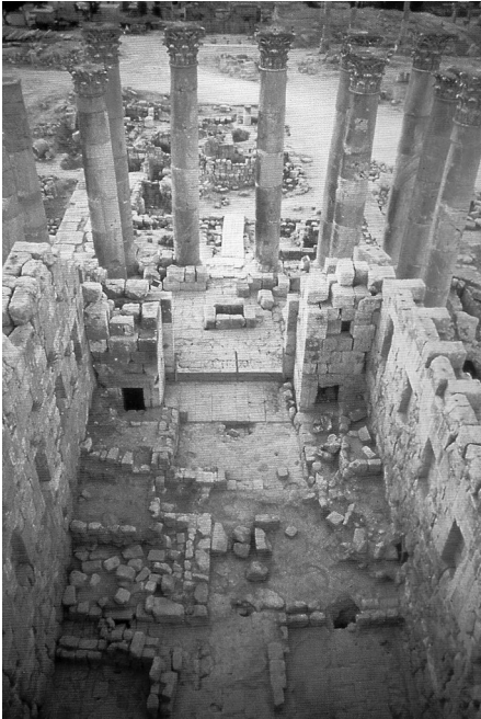
Fig. 12. Gerasa, general view of the cella of the Temple of Artemis, facing east (after Parapetti 2002: Fig. 45).
